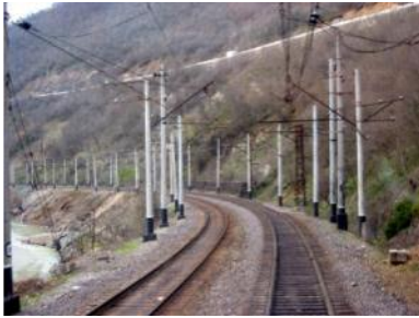
3kV-DC Overhead Catenary, Georgia
